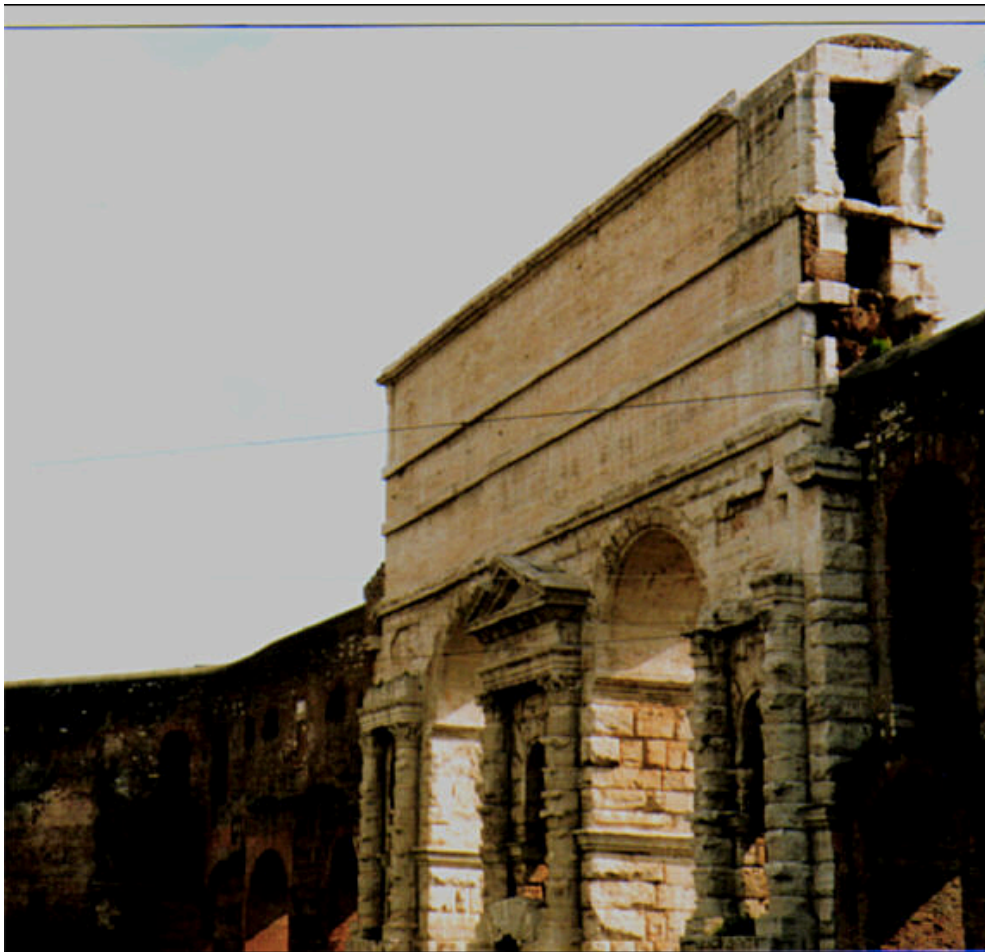
Remains of the Aqua Claudia in Rome; water flowed through the channels near the top of the structure. Wikimedia , Diana, GFDL or CC-BY-SA-3.0
